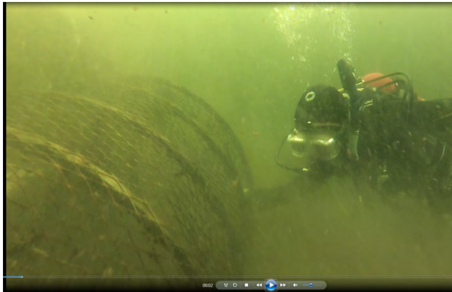
Figure 4-3. Example of diver cleaning the existing intake
